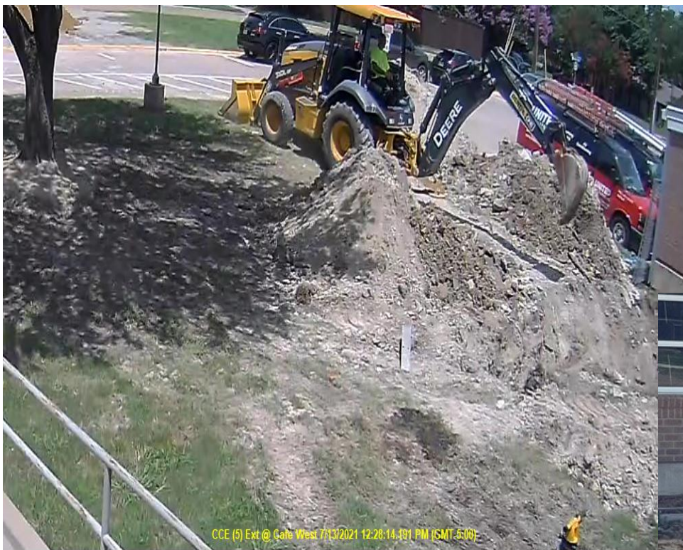
CCE – GREASE TRAP REPLACEMENT
